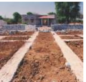
Foundation of the Third Classroom Block 1996
