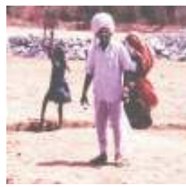
Breaking earth for the first block - Contractor Narayan ba, 1992
